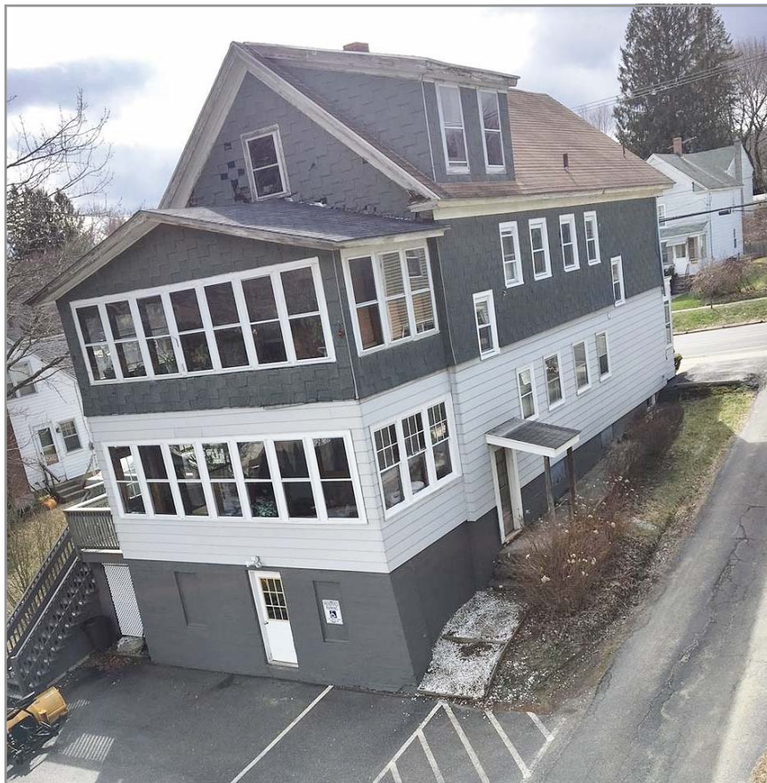
DUPLEX (TWO UNITS) — 316 ONOTA STREET
